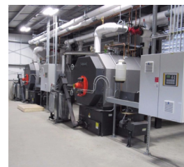
A biomass thermal system can provide hot air, water, and process heat
